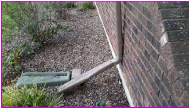
ideally drains 6 feet from foundation
